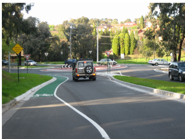
Figure 1: Good practice example of a roundabout in Melbourne
