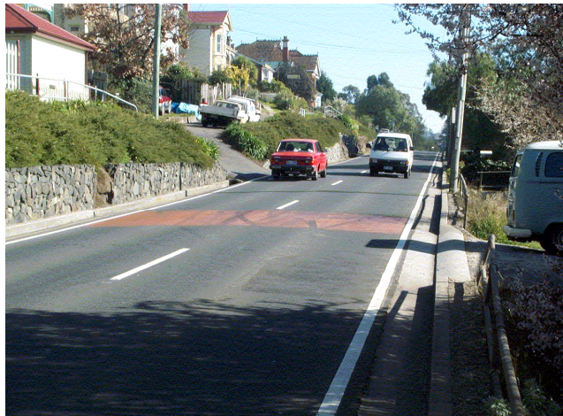
‘Figure 3 – Flush pavement bands in Launceston’
