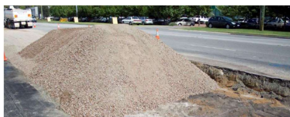
City of Canning – Upgrade of Welshpool Road using C&D material as road base and sub base
