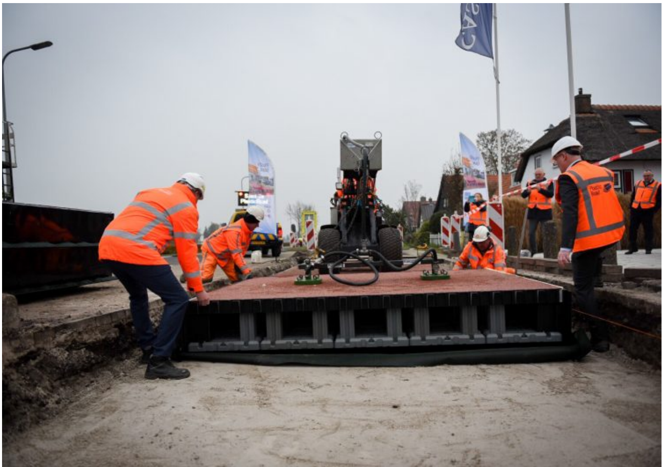
Figure 5.3: Second trial of PlasticRoad in the Netherlands
